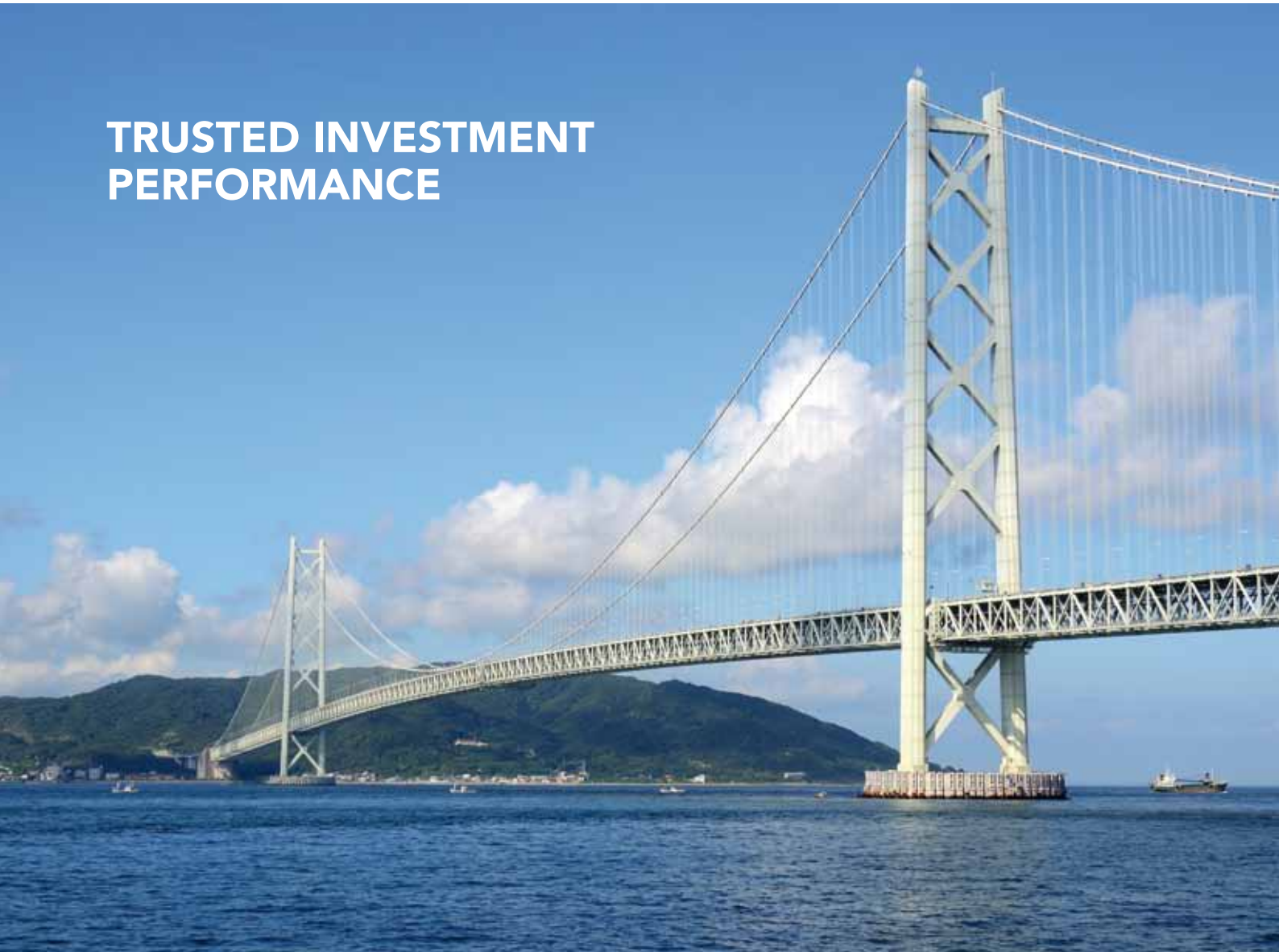
Akashi Kaikyō Bridge, Japan. Longest suspension bridge in the world, with a central span of 1 991 metres.
